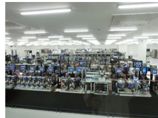
Clean room with latest air-conditioning system
